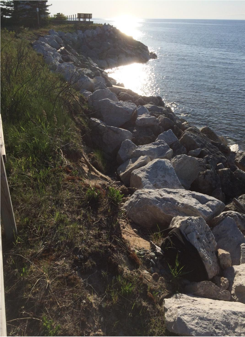
Settling of Erosion Control Rock East of Lighthouse
