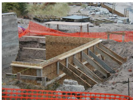
Foundation Forms Being Constructed
