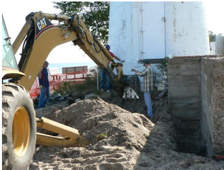
Construction begins as sand is removed for the foundation
