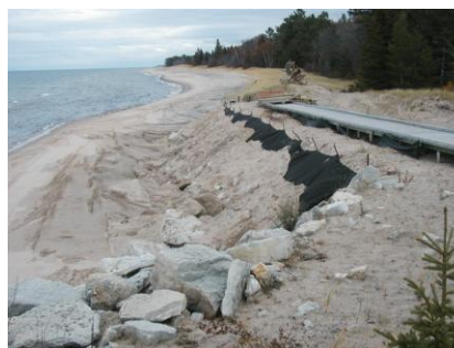
Temporary repair work to sand bank east of the lighthouse
