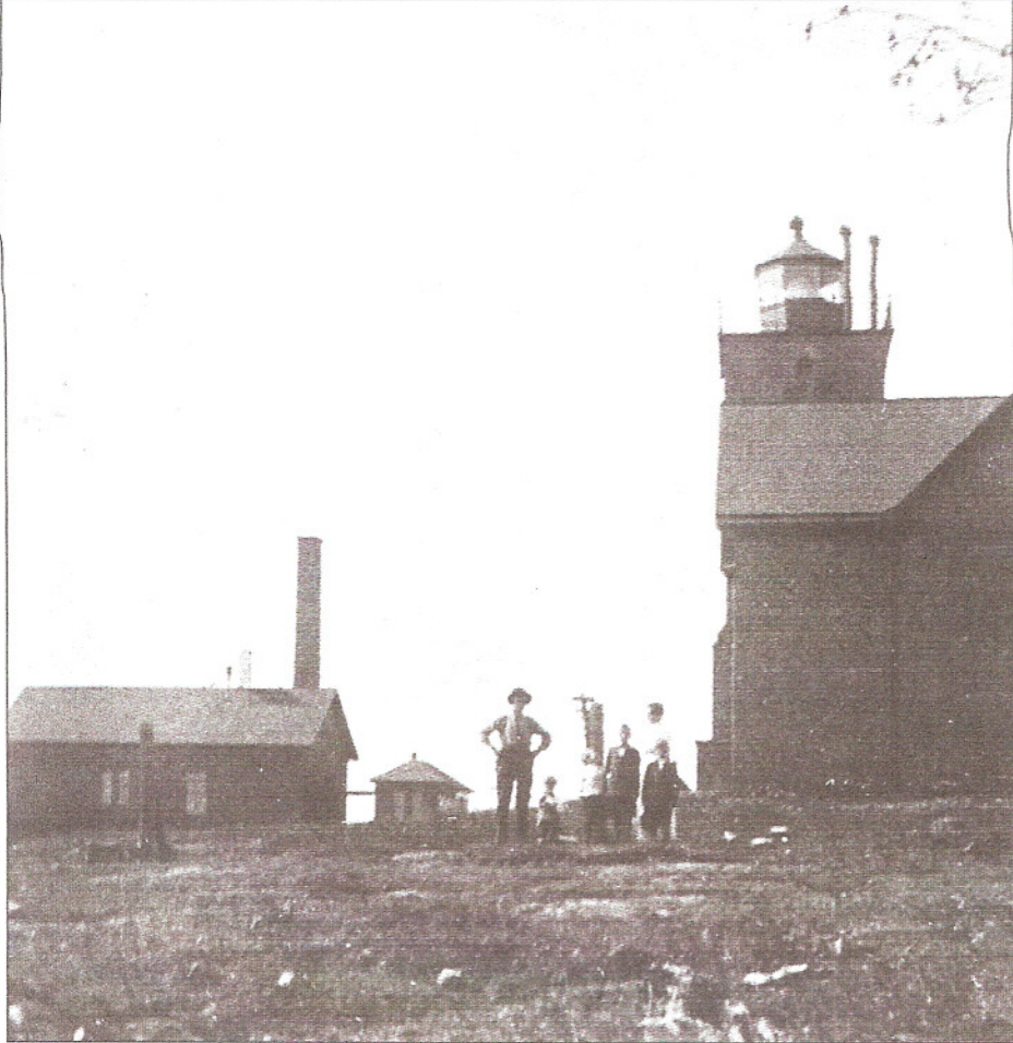
The Singleton family at the Two Harbor Light Station. Note the whistle fog signal, left of the chimney of the building at left. Small building is the oil house.
