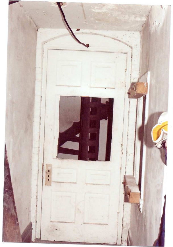
The original wooden door at the base of the tower.
